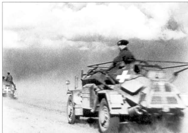
The light four wheeled armored cars of the Sd.Kfz.221-223 series were more common. They were fast and maneuverable with good cross country performance and were easy to service. Here we see a leichte Panzerspähwagen (Fu) (Sd.Kfz.223), identifiable by its folded down frame antenna, traveling at high speed down a dusty country road in Poland in late September 1939. Markings include a white national cross painted on the side of the hull and rear radiator grille. Though not clear in the photo, it also has the standard Wehrmacht vehicle registration plate mounted on both rear mudguards.
