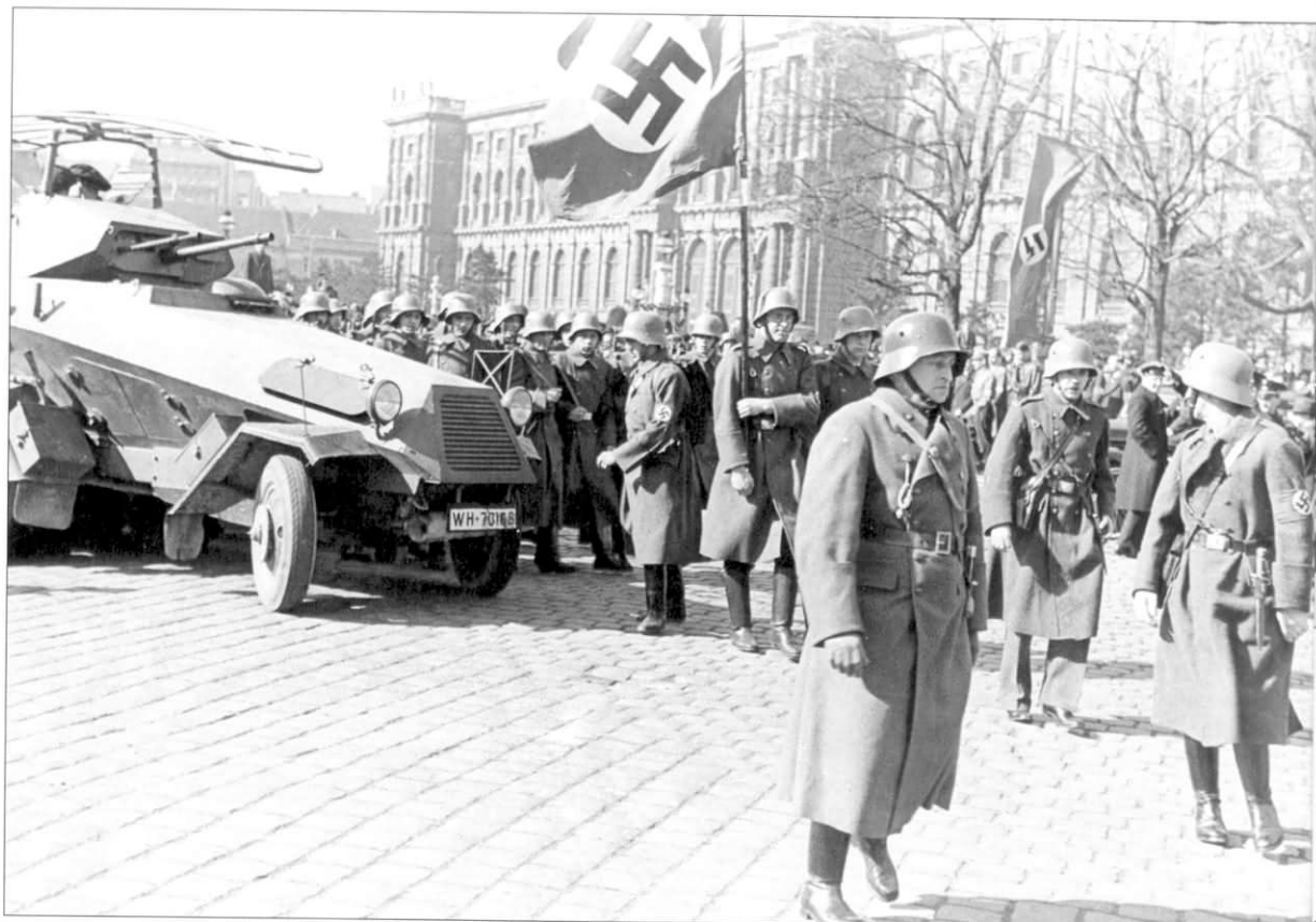
A schwere Panzerspöswagen (Fu) (Sd.Kfz.232) of 2. Panzer-Division takes part in a parade in Vienna in the spring of 1938. One of the earliest armored cars of this type, 123 were manufactured from 1932 to 1937 in this and the standard Sd.Kfz.231 variation. The Sd.Kfz.232 can be identified by the large frame antenna that pivoted above the turret. The Sd.Kfz.263 was similar except that it had a fixed turret with a single MG13 and the shape of the antenna display was different, being supported by two legs directly off the turret. Typical for prewar vehicles, no national markings have been applied and only the standard license number plate, 'WH-70168', is visible.
