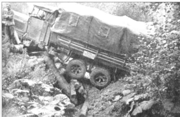
A primitive bridge has collapsed under the weight of this Henschel 33D1 truck. The roads in Poland were mainly constructed for horse drawn transport and such occurrences were not uncommon during the German Army's advance.
