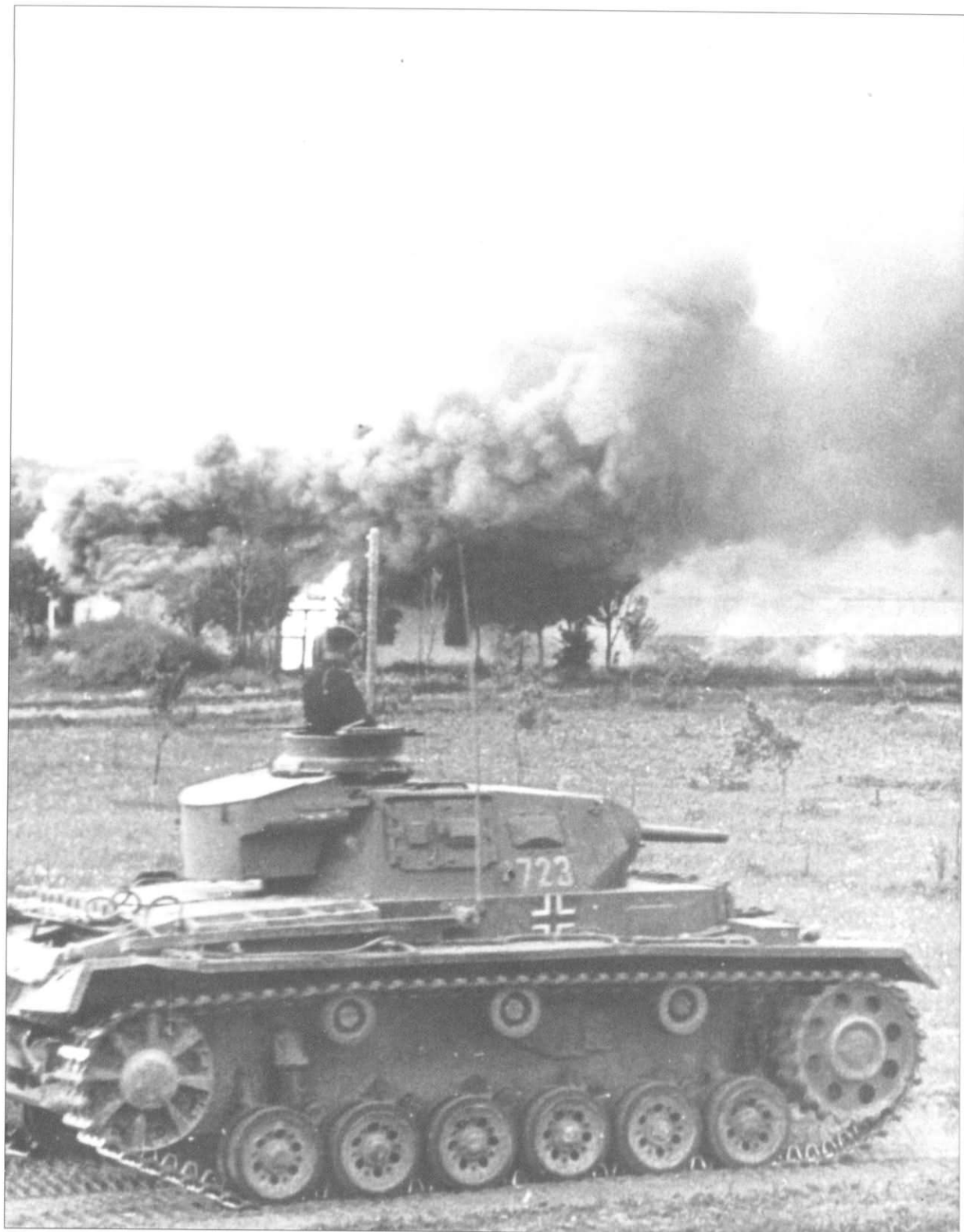
A Pz.Kpfw.III Ausf.E passes the same farmhouse. The tactical number '723', painted in yellow, is plainly visible on the side of the turret, as is the black and white national cross on the side of the hull. Turret stowage bins were introduced on the Ausf.G but were fitted to many early vehicles in the field workshops.
