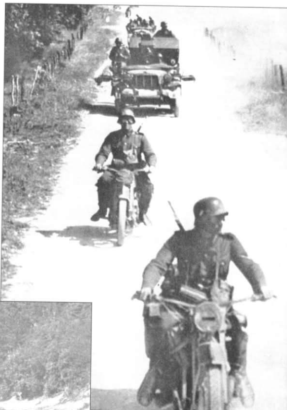
Two motorcycles lead a column of vehicles across the French countryside, including Sd.Kfz.10/4 armed with the 2cm FlaK30 FlaK38 anti-aircraft gun. In addition to its anti-aircraft duties, the FlaK30/38 was also used against light armored targets on the ground using armor piercing ammunition. Later models were provided with an 8mm armored cab.
